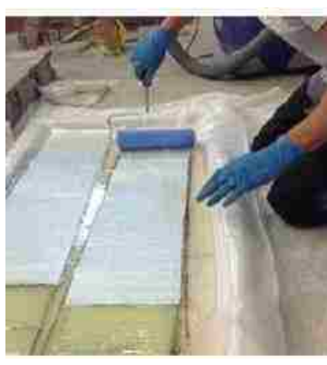
Saturate fiber in epoxy
