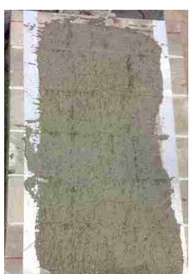
Apply matrix on wall
