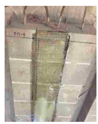
Apply saturated sheet on wall
