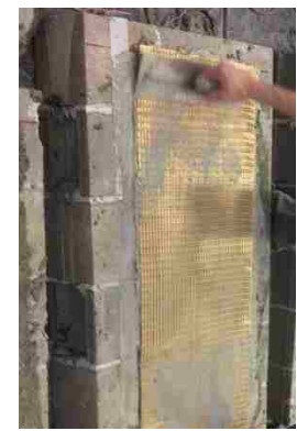
Apply fiber on matrix
